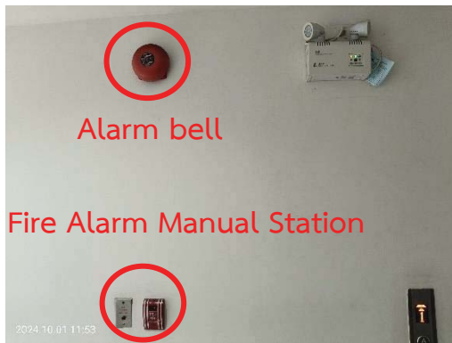
Alarm bell & Fire Alarm Manual Station
